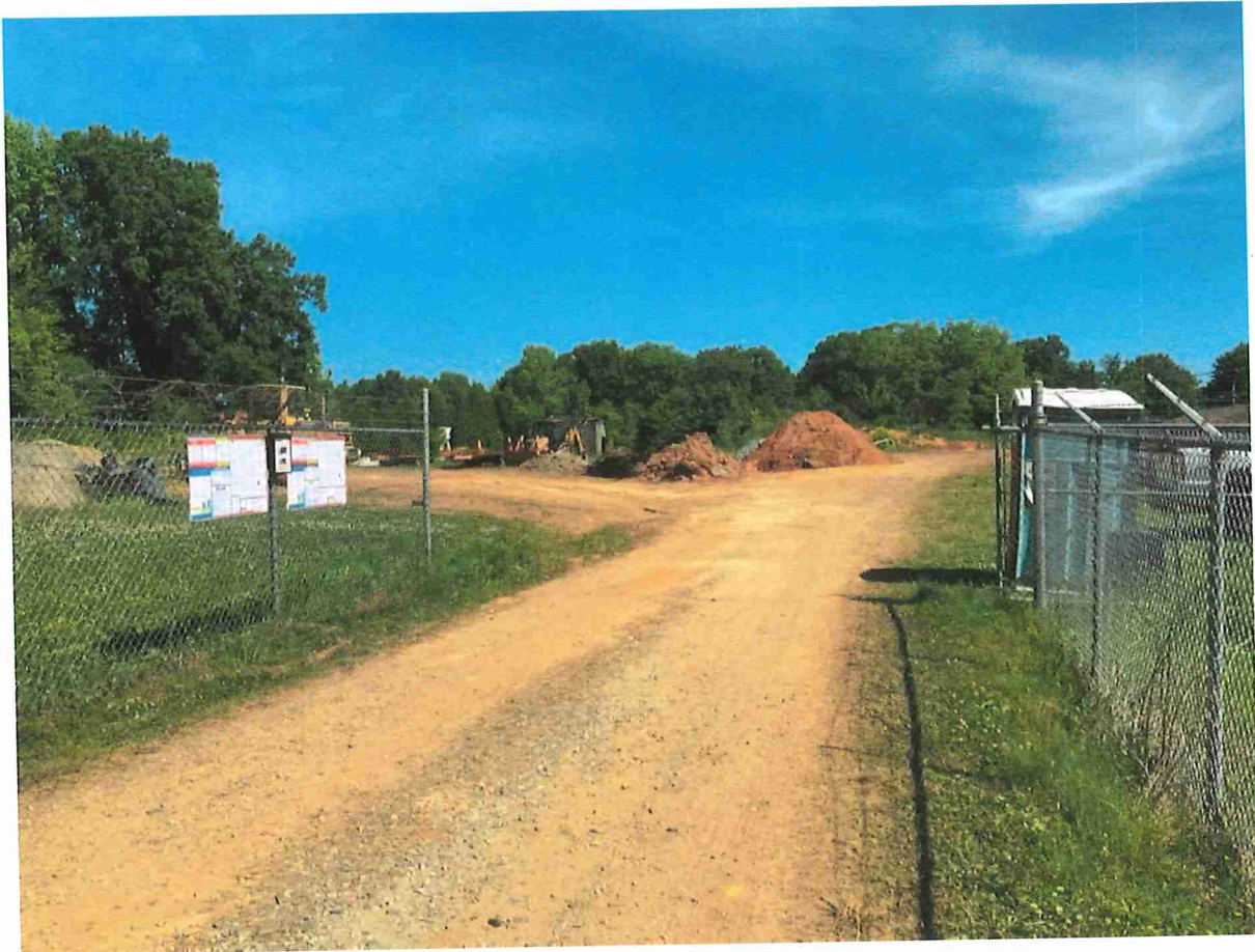
Pictures during construction of the sewer line work summer 2021
